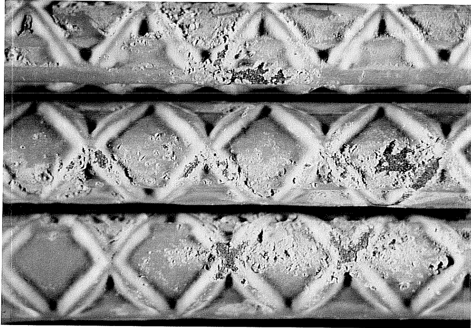
Figure 4.13 Damage due to vibration on #4 bars – slab specimen.
