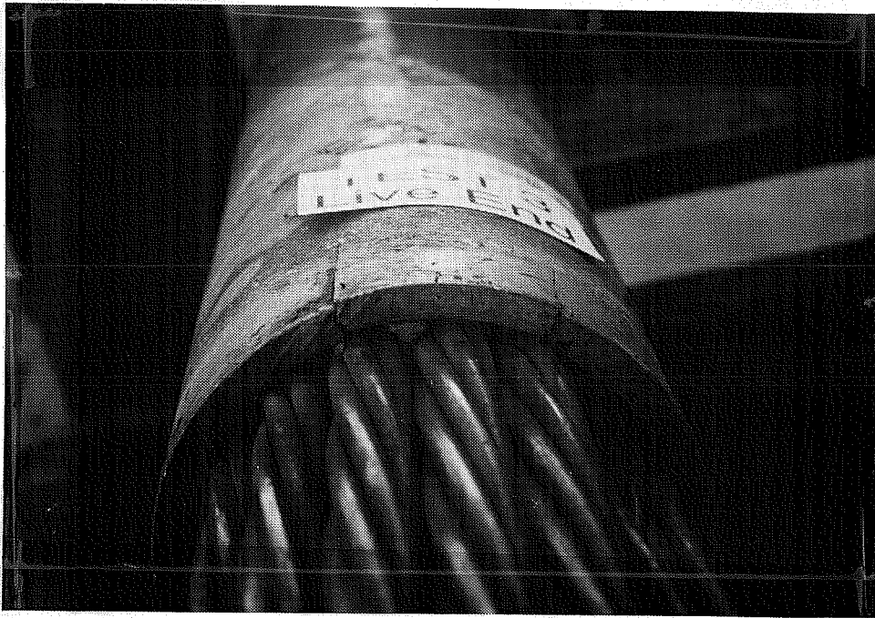
Figure 4.34 End view of the cracking of the outside end of a Test #3 deviator duct.
