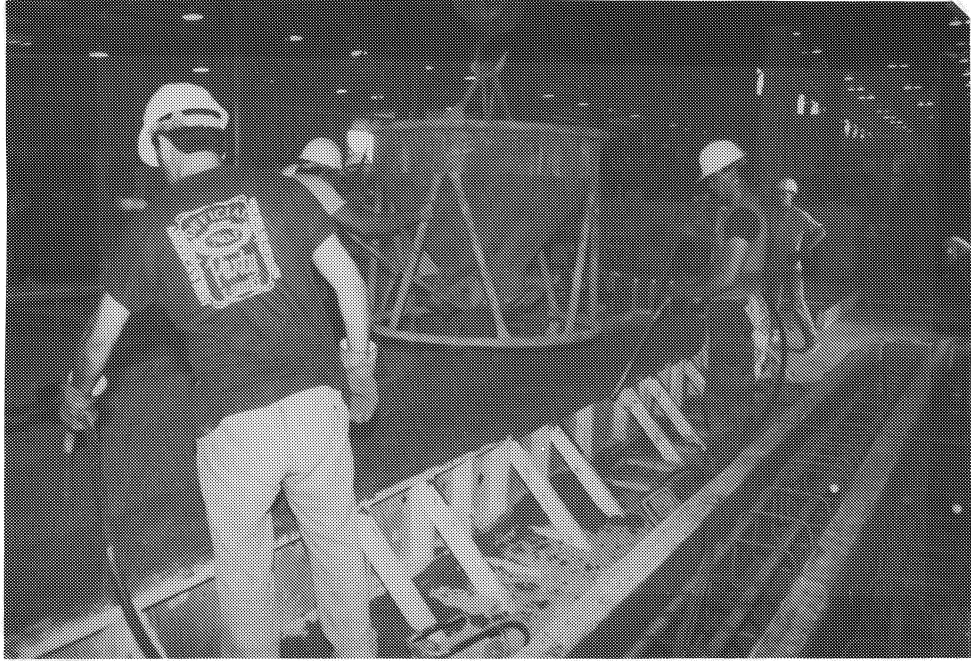
(a) Concrete placement and compaction
