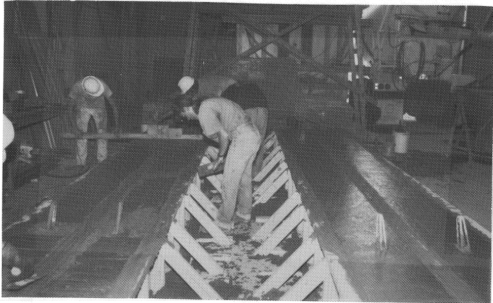
(b) Screeding and trowelling the beam surface
