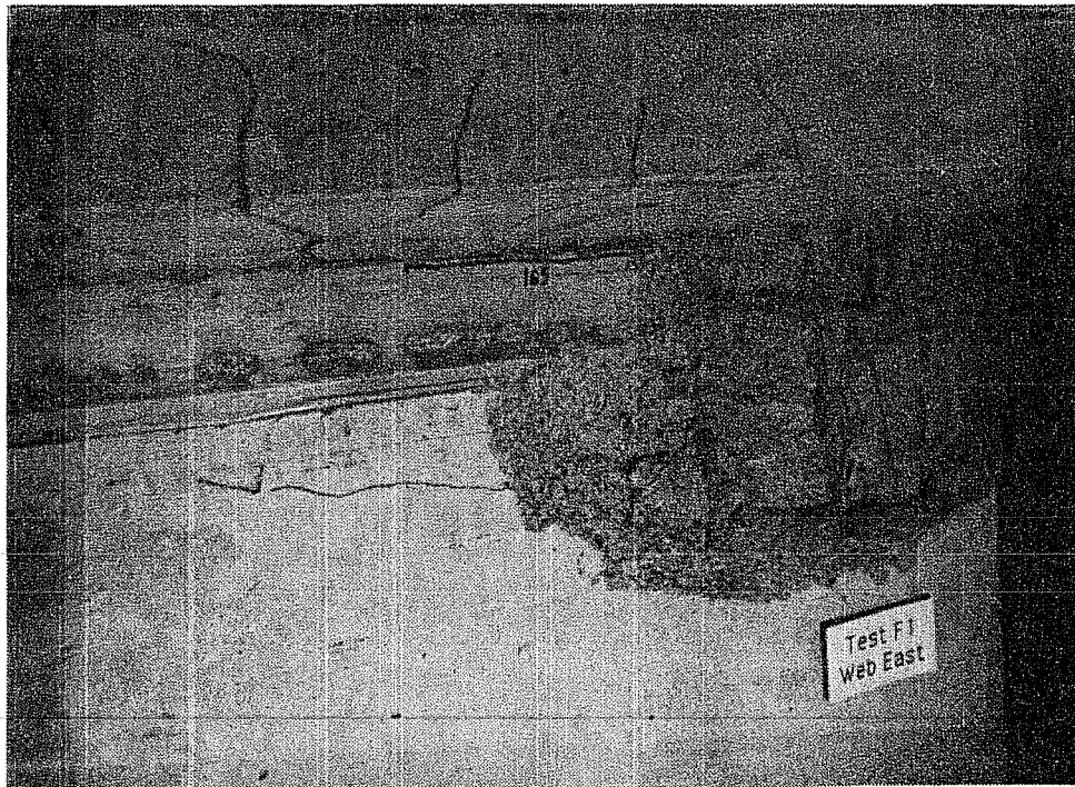
Figure 137 Anchorage "A" failure and flange bottom face cracking, Specimen F1.
