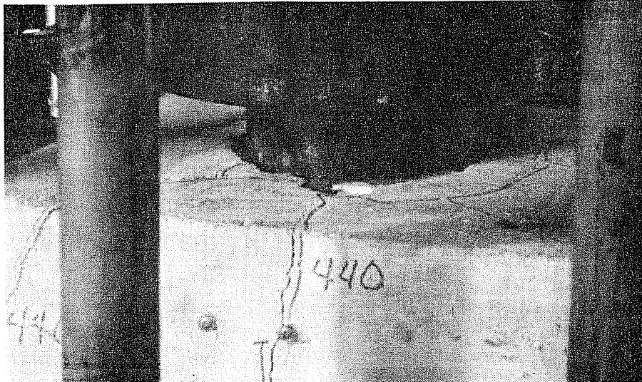
Figure 28 Specimen MP-B anchorhead at failure.
