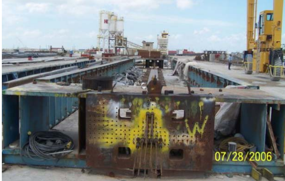
Figure 3-9: Prestressing bed at HEI Corpus Christi Plant (photograph courtesy of Chris Leonard)
