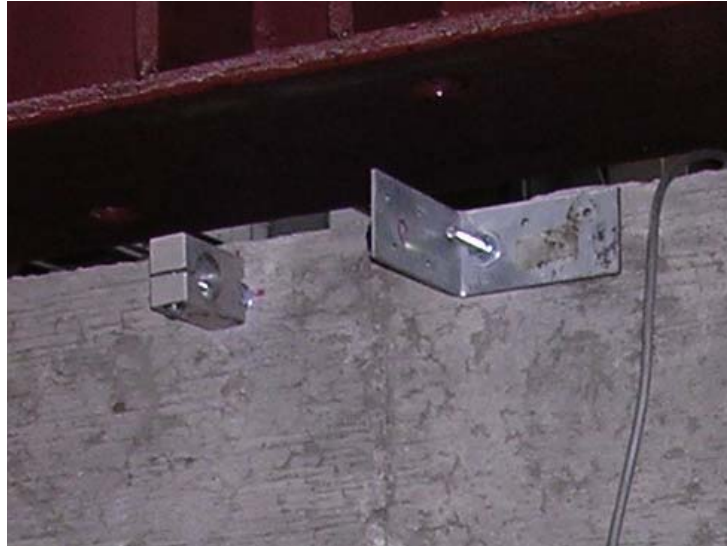
Figure 4-6: Aluminum clamp and angle before DCDT installation
