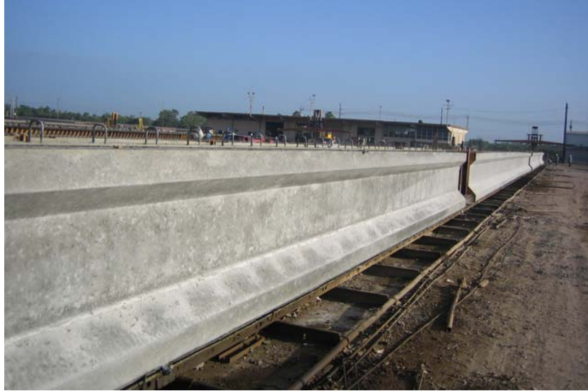
Figure 6-5: Line of Type-IV girders after release at TCC Victoria plant
