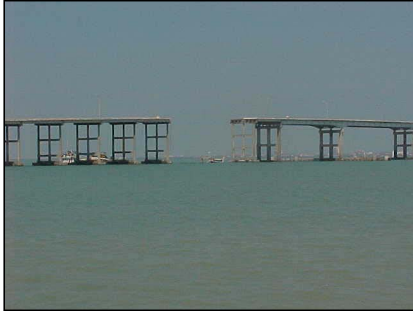
Figure 1.2: The Collapsed Portion of the Queen Isabella Causeway (Source: South Texas Business Directory).
