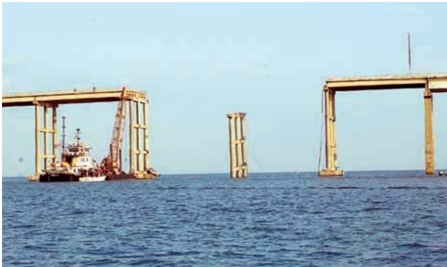
Figure 1.1: Queen Isabella Causeway Damage
