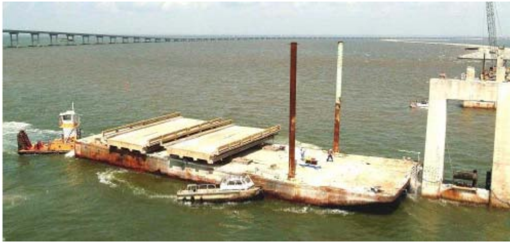
Figure 1.3 Florida DOT's impact test on Causeway pier to be demolished
