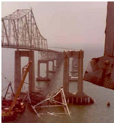
Figure 1.1 Aftermath of the 1980 Sunshine Skyway Collapse
