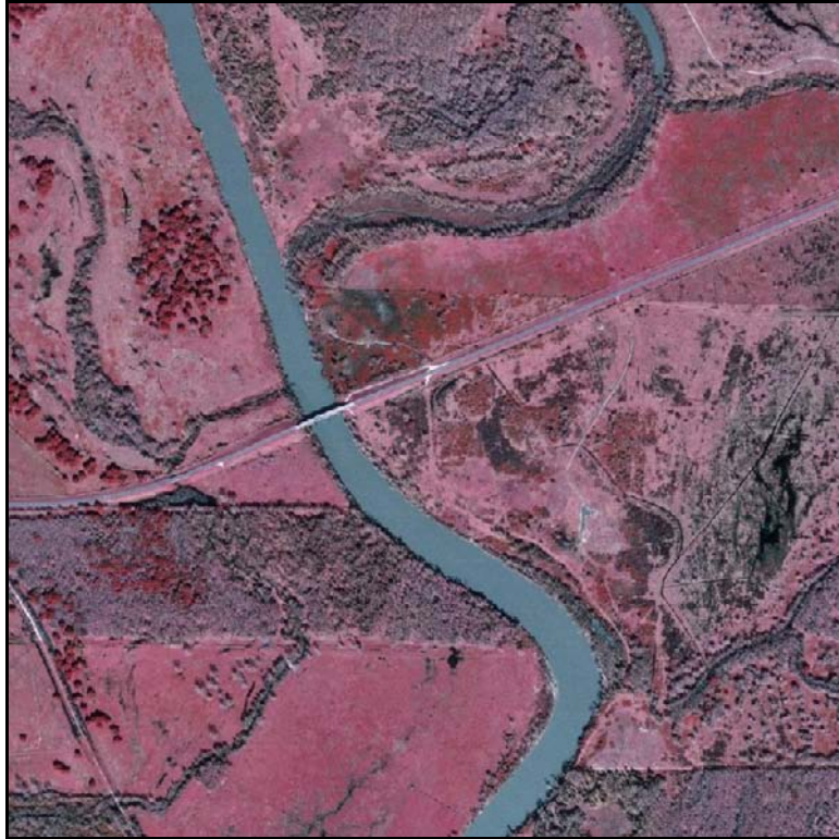
Figure 5.2: Satellite Image of the Colorado River – FM 521 Bridge and the Surrounding Region of Interest.
