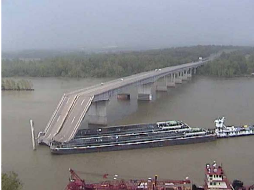
Figure 1.2: Webbers Falls, OK I-40 Bridge Damage
