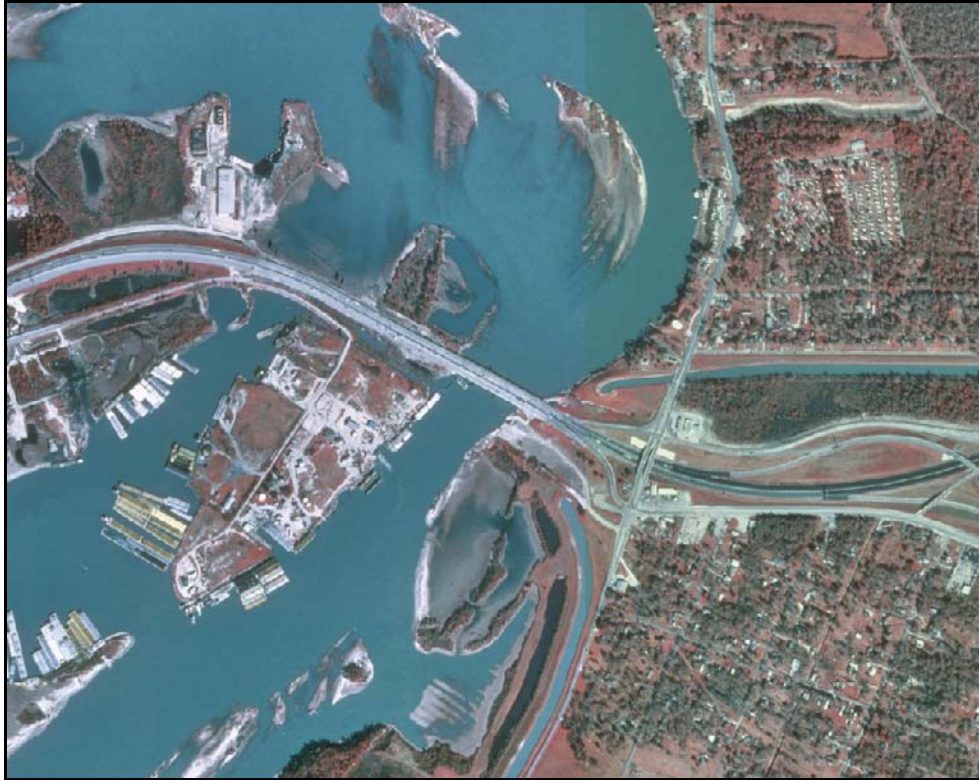
Figure 5.7: Satellite View of the San Jacinto River – IH 10 Bridge
