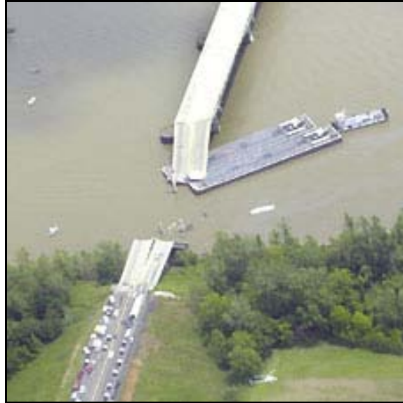
Figure 1.3: Bridge in Webbers Falls Oklahoma Collapses Due to Vessel Collision (Source: The Anniston Star).
