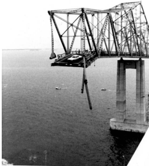
Figure 2.2: Sunshine Skyway Damage
