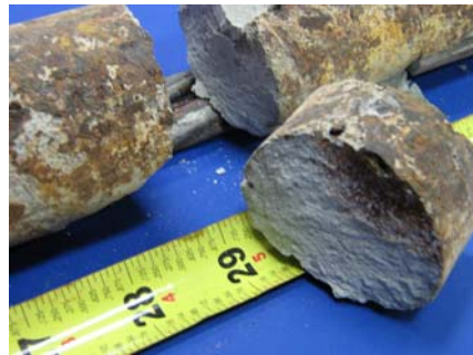
South Duct Grout
