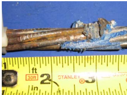
South Duct Strand (Coating Removed)
