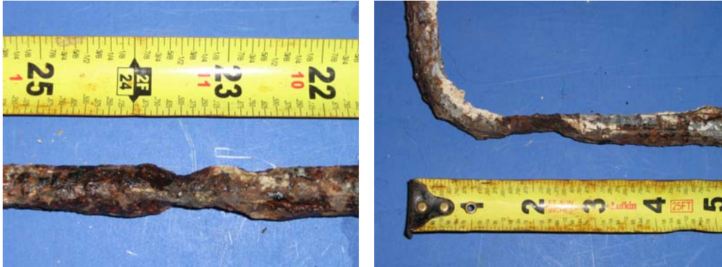
Figure 5.12: Beam 1.2 Autopsy Elements-Longitudinal Bar (Left) and Stirrup (Right)
