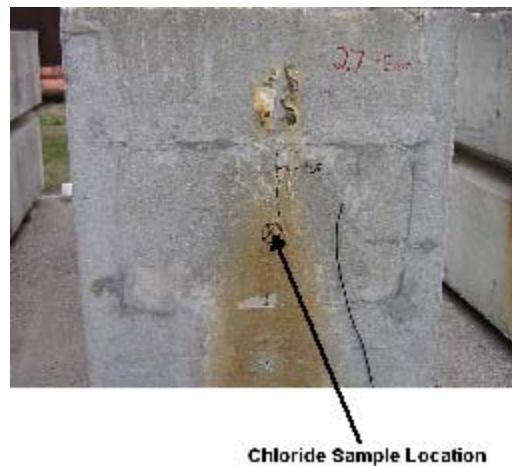
Figure 3.8: Chloride Sample Location for Anchorage Exposure Specimens
