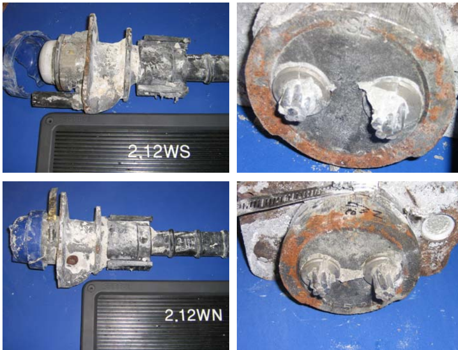
Figure 5.61: Beam 2.12 West End Anchorages (Control End)-South Duct Anchorage (Top, Left and Right) and North Duct Anchorage (Bottom, Left and Right)
