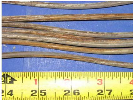
South Duct Strand
