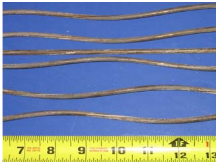
South Duct Strand
