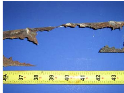
Top of North Duct
