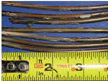
North Duct Strand (Coating Removed)
