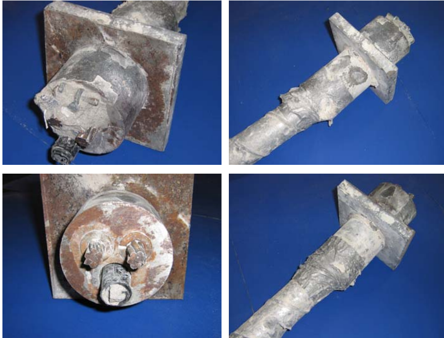
Figure 5.51: Beam 2.9 East End Anchorages (Dripped End)-North Duct Anchorage (Top, Left and Right), and South Duct Anchorage (Bottom, Left and Right)
