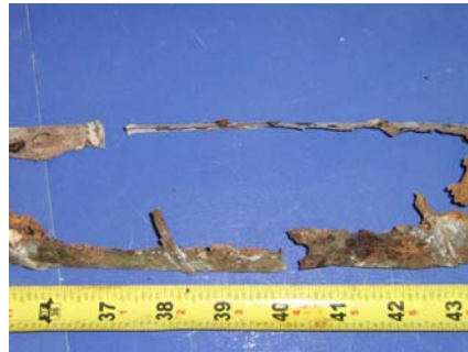
Top of North Duct
