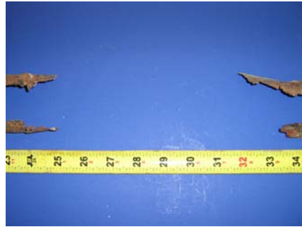
South Duct (Top Half)
