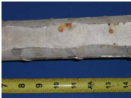
South Duct Grout
