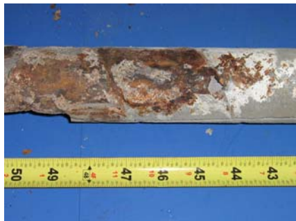
South Duct Grout
