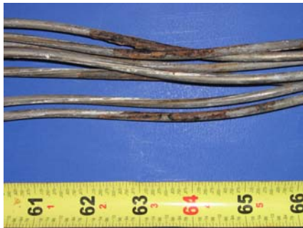
South Duct Strand
