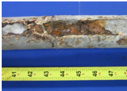
South Duct Grout
