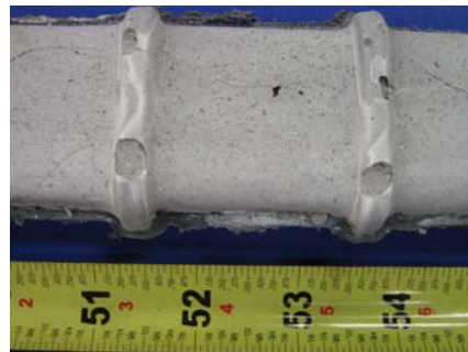
North Duct Grout
