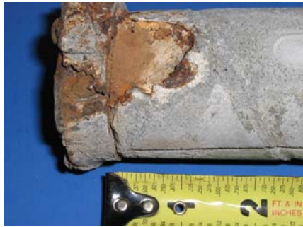
South Duct Grout
