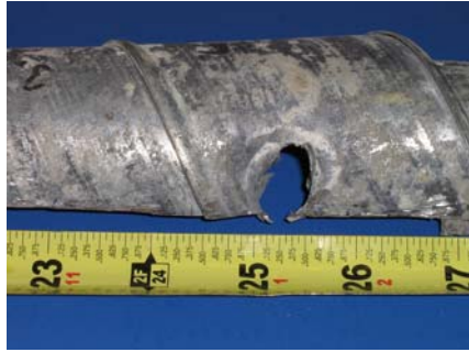
Top of North Duct
