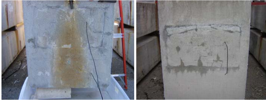
Figure 5.60: Beam 2.12 Anchorage Zones: East End Anchorage With Dripper (Left) and West End Anchorage Without Dripper (Right)
