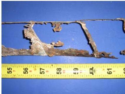
Top of South Duct
