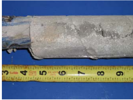
South Duct Grout
