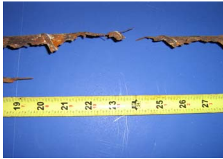
Top of South Duct
