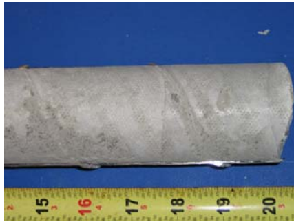
South Duct Grout
