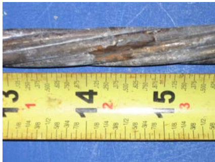
South Duct Strand
