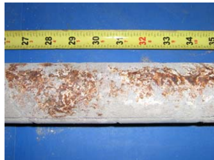
North Duct Grout
