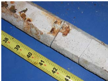
South Duct Grout
