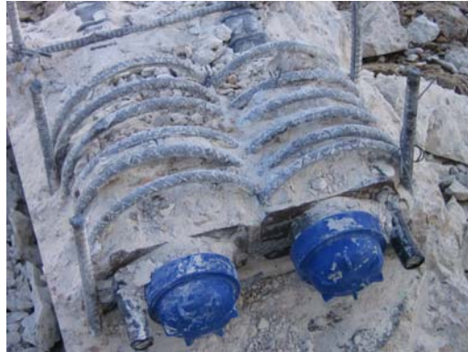
Figure 5.4: Removal of Post-Tensioning Anchorages (East End Anchorage of Beam 2.12 pictured)
