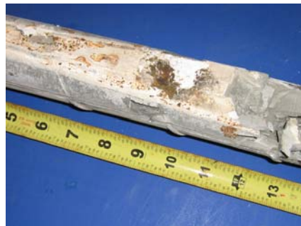
North Duct Grout
