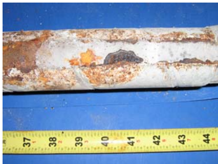
South Duct Grout
