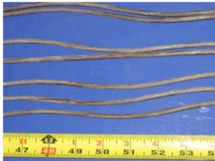
South Duct Strand
