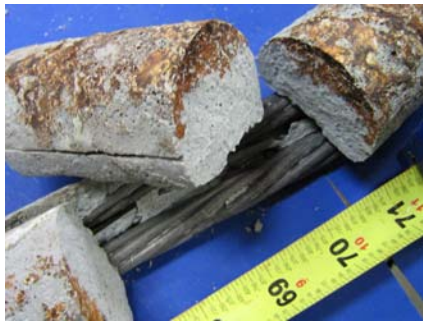
North Duct Grout
