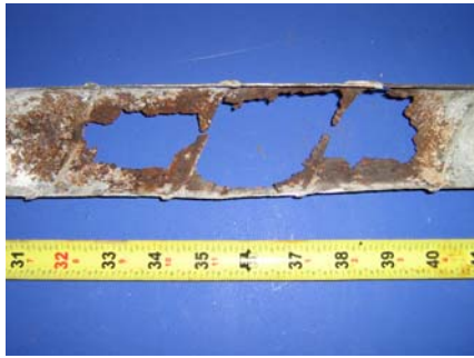
Top of North Duct
