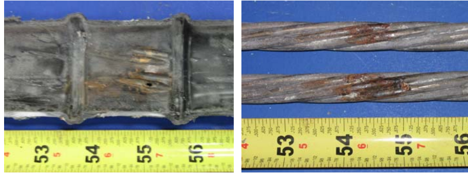
Figure 5.59: Beam 2.12-Abrasion Damage to Interior of North Duct (Left) and Strand from Same Location (Right)
