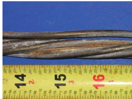
North Duct Strands
