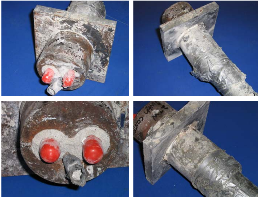
Figure 5.37: Beam 2.7 West End Anchorages After Removal (Controls): North Duct Anchorage (Top, Left and Right), and South Duct Anchorage (Bottom, Left and Right)
