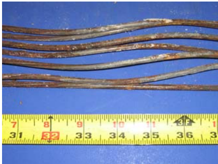
South Duct Strand
