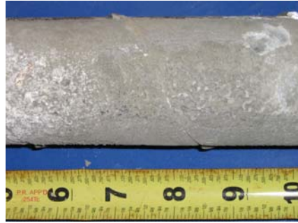
North Duct Grout
