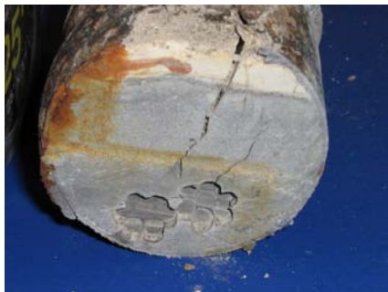
South Duct Grout
