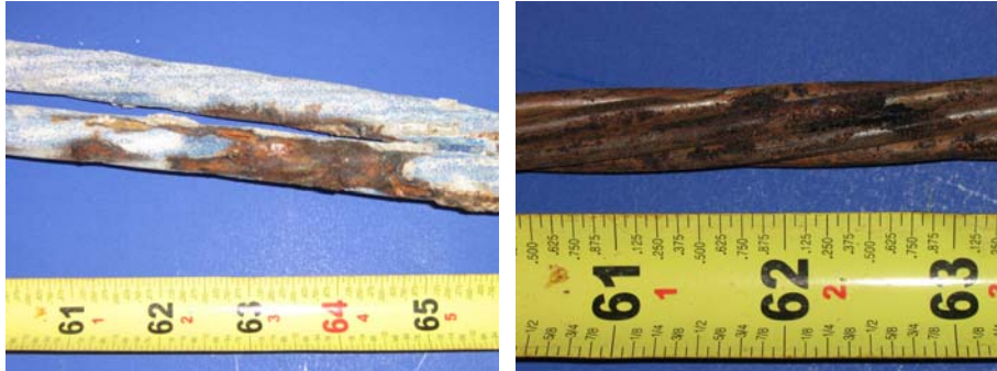
Figure 5.33: Beam 2.7-South Duct Strand with Coating (Left) and After Removal of Coating (Right)
