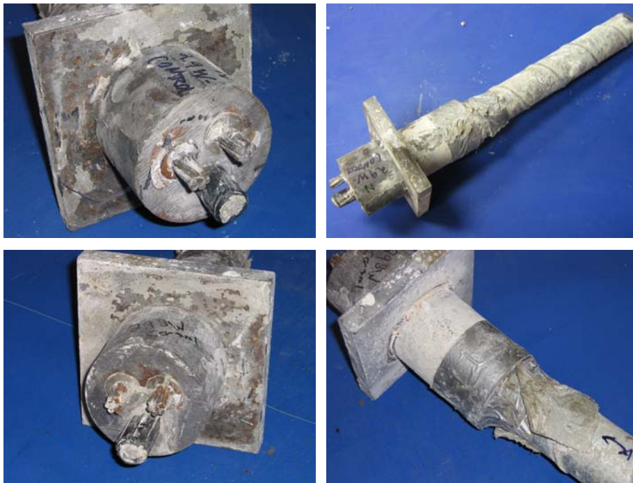
Figure 5.49: Beam 2.9 West End Anchorages (Controls) After Removal-North Duct Anchorage (Top, Left and Right), and South Duct Anchorage (Bottom, Left and Right)
