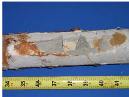
North Duct Grout
