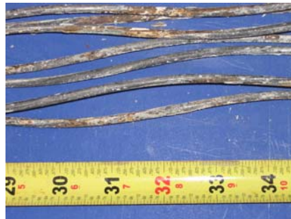
North Duct Galvanized Strand
