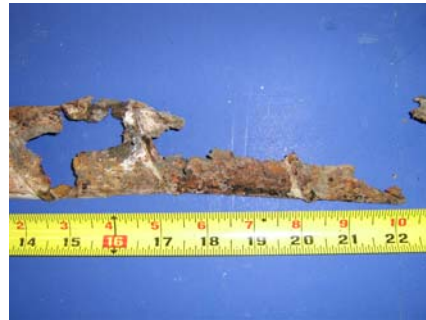
Top of North Duct
