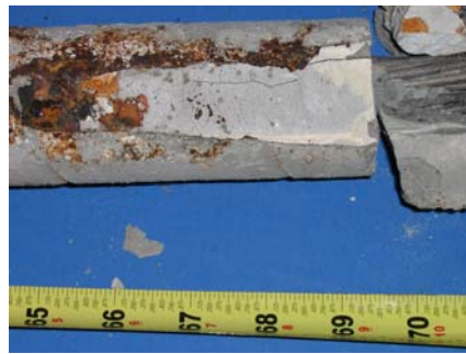
North Duct Grout
