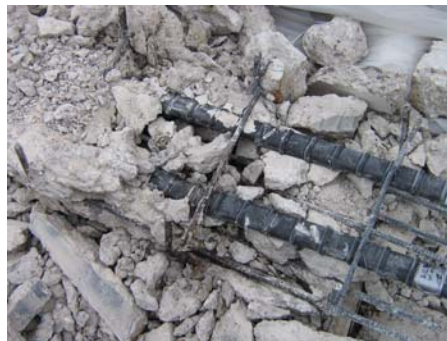
Figure 5.58: Beam 2.12 During Autopsy
