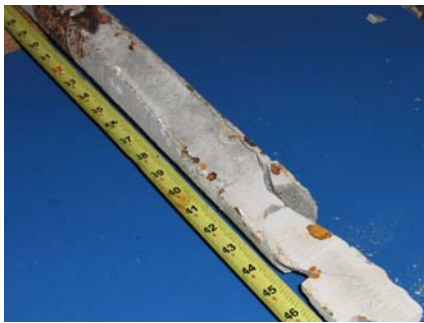
South Duct Grout
