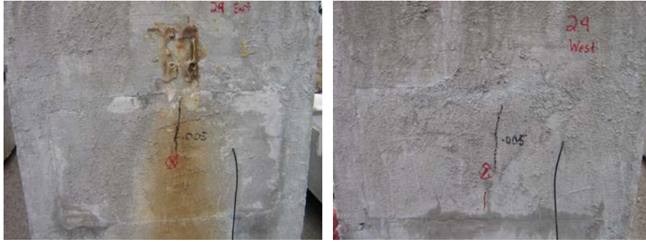
Figure 5.48: Beam 2.9 Anchorage Zones-East End (Left) with Dripper, and West End (Right) Without Dripper
