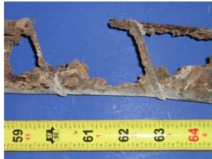
Top of North Duct
