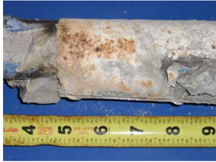
North Duct Grout
