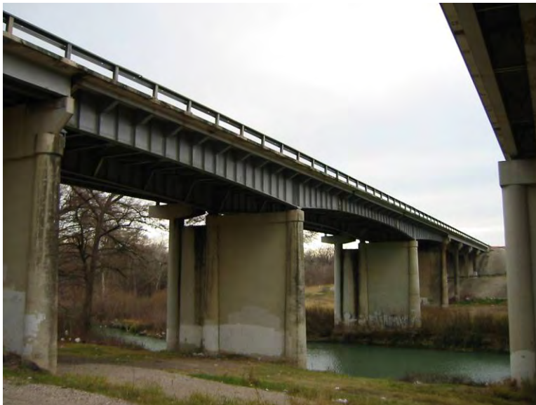
Figure 3.2 Center Three Spans of Medina River Bridge (viewed from North)
