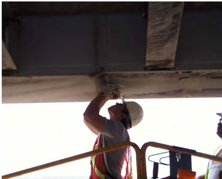
Figure 5.4 Installation of Strain Gage near Transition in Flange Thickness
