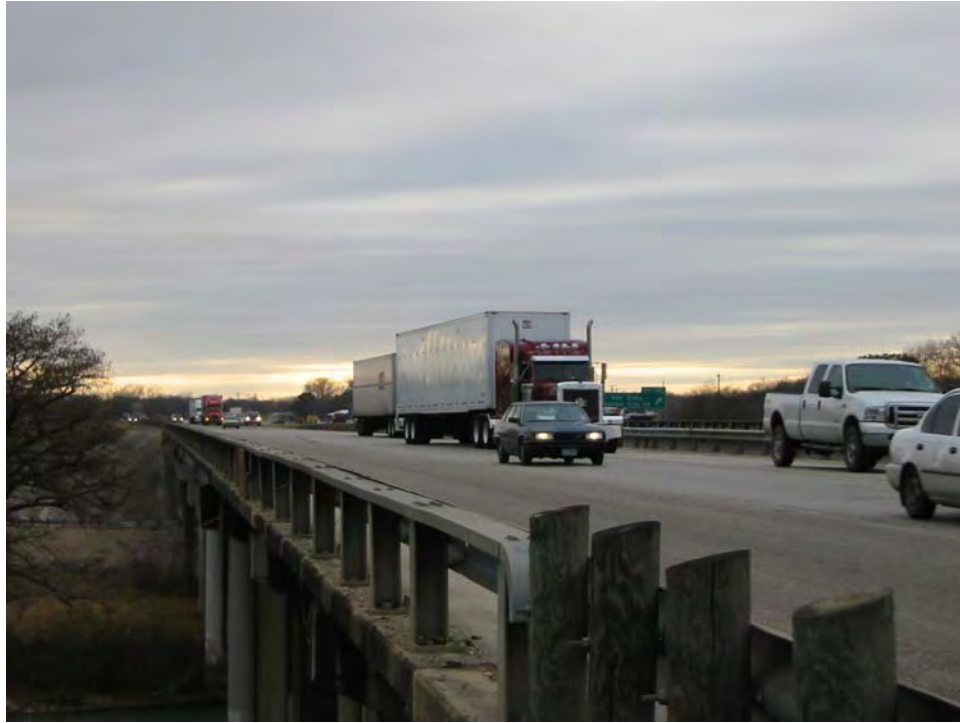
Figure 4.3 Observed Traffic Patterns on Medina River Bridge
