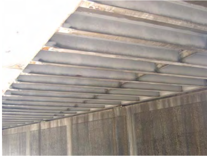
Figure 3.23 Elastomeric Bearings above Skewed Abutment
