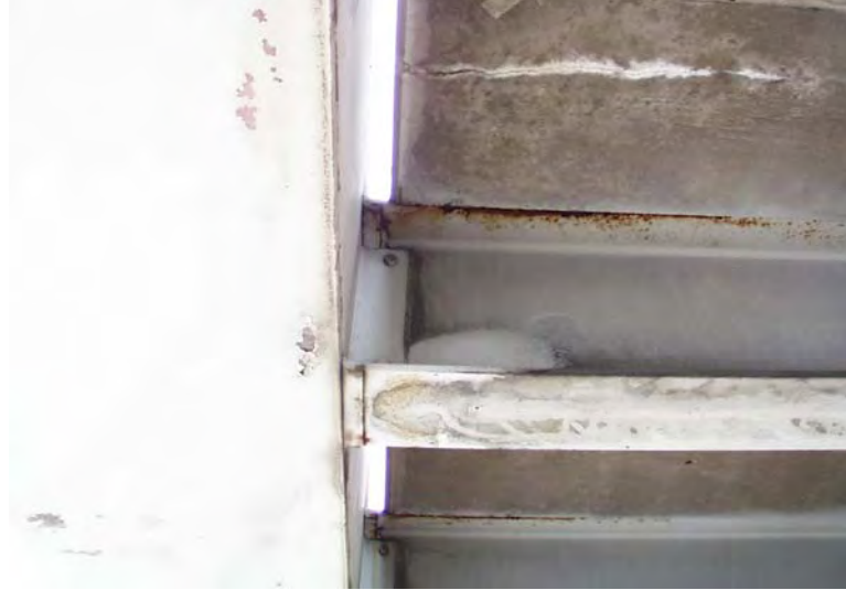
Figure 3.20 Welded Connections between Floor Beams and Longitudinal Box Girders
