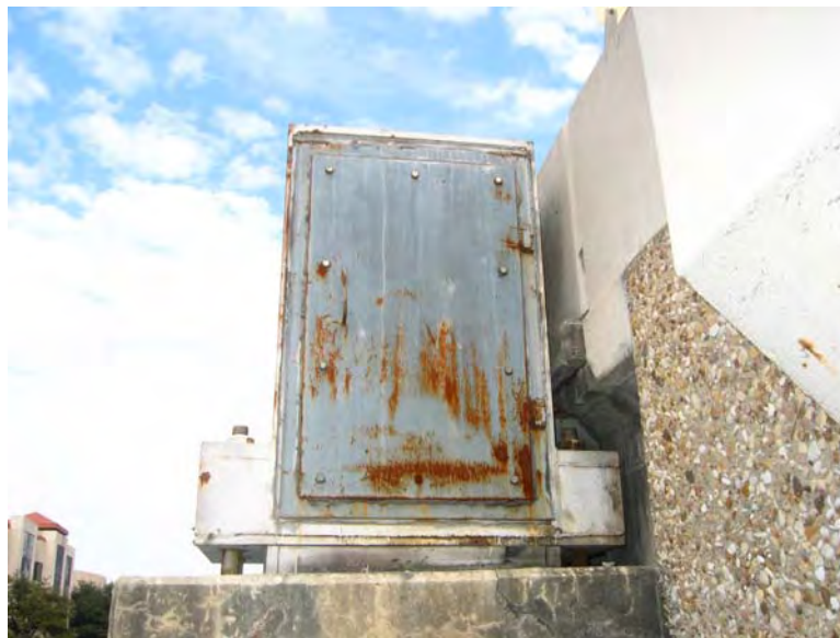
Figure 3.22 Elastomeric Bearing at South End of West Girder
