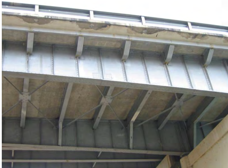
Figure 3.9 West Girder of Medina River Bridge
