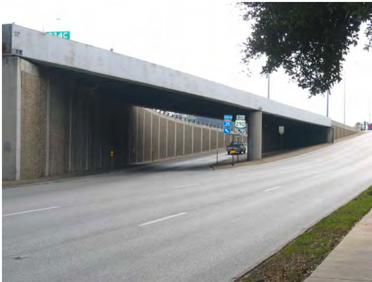
Figure 3.17 12 th Street Exit Ramp Crosses Grade-Level Entrance Ramp to I-35
