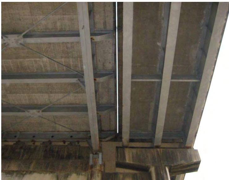
Figure 3.4 Separation between Original Structure and Lane Added in 1971
