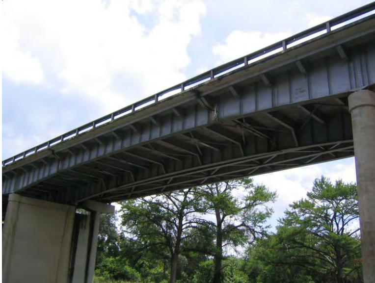
Figure 3.3 Center Span of Medina River Bridge (viewed from South)
