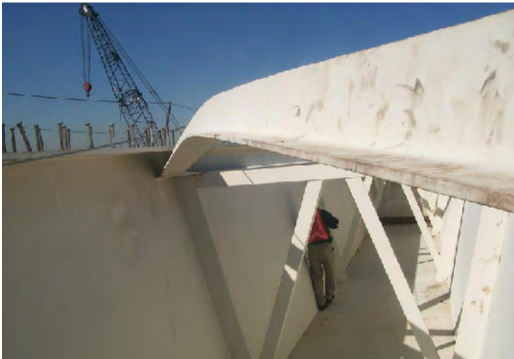
Figure 1.7: Trapezoidal Box Girder Failure during Construction (T. Helwig, U. of Houston)
