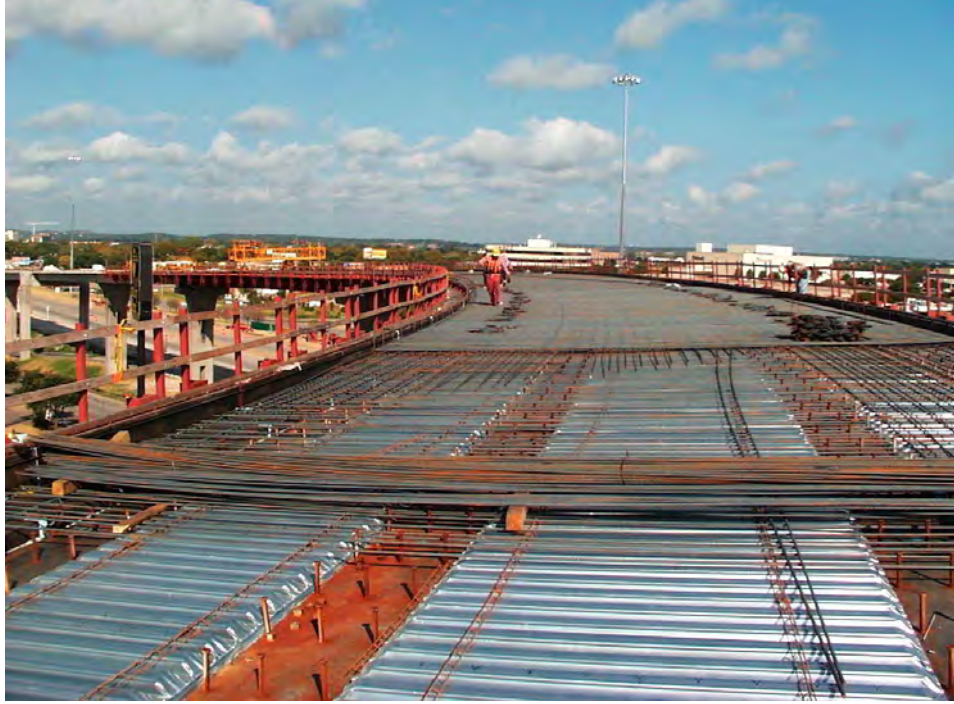
Figure 3.4: Deck Forms and Reinforcement Installation
