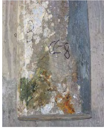
Moisture under the wrap over bottom region of rebar B.
