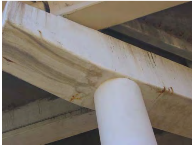
Figure 4.3 Rust staining on bent
