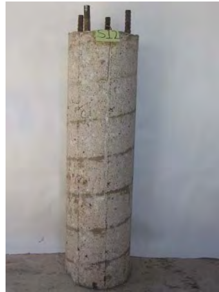
Specimen S12 after removal of wrap.
