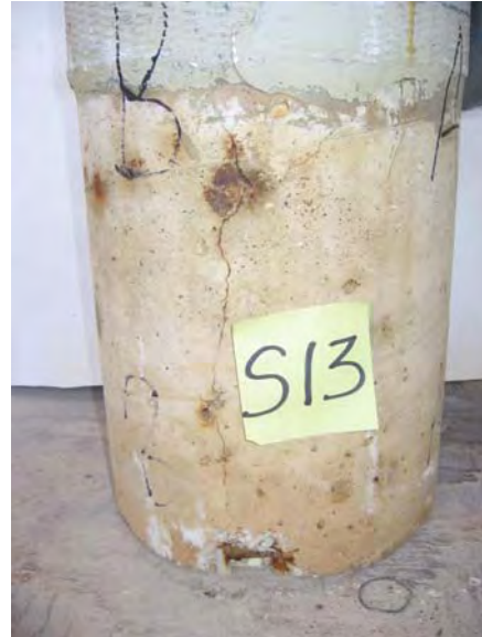
Crack and rust stains over rebar B on cylinder S13.
