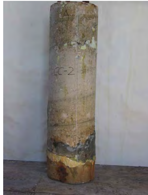
Repair patch and rust stain over rebar B.
