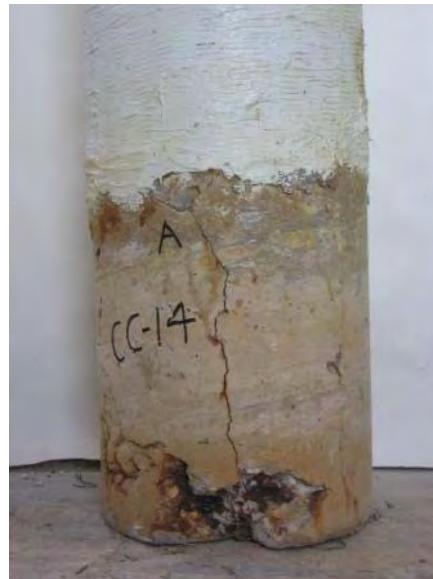
Vertical crack over rebar A with spalled-off section.
