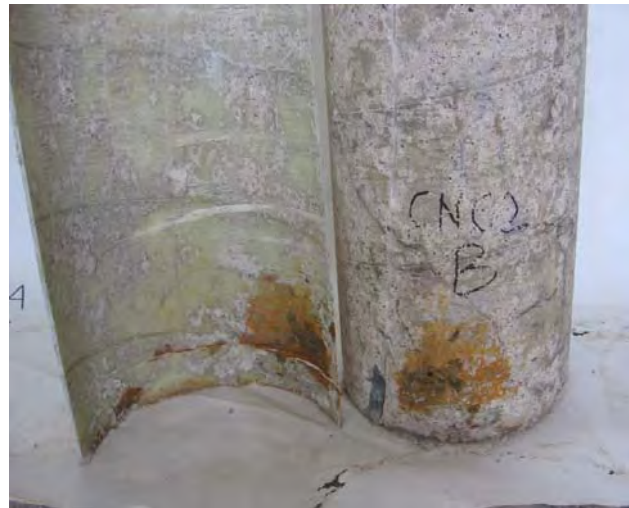
Cylinder CNC2, after removal of wrap with a large rust stain over rebar B.
