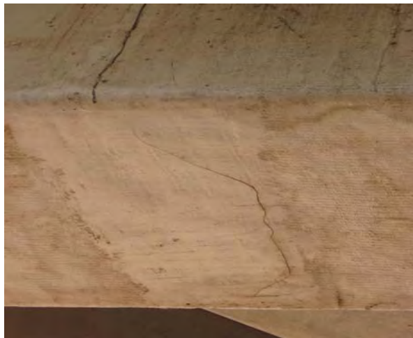
Figure 4.6 Crack on underside of bent on Structure 5
