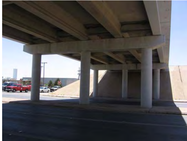
Figure 4.11 US 87 over 82 nd St.
