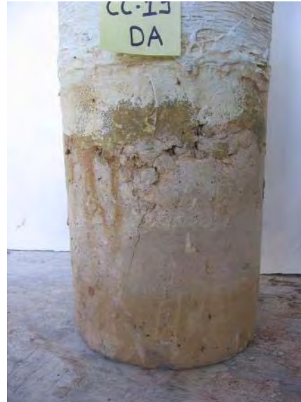
Area DA just below wrap edge was not consolidated properly. Repair patch visible at the bottom.
