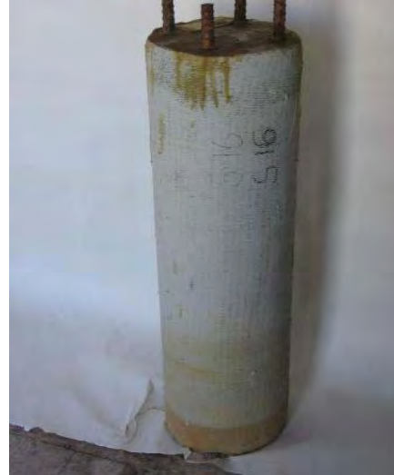
Cylinder S16 completely wrapped.
