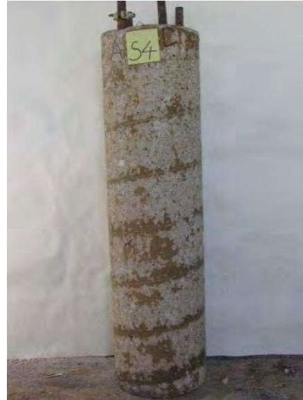
Column S4 after removal of wrap.
