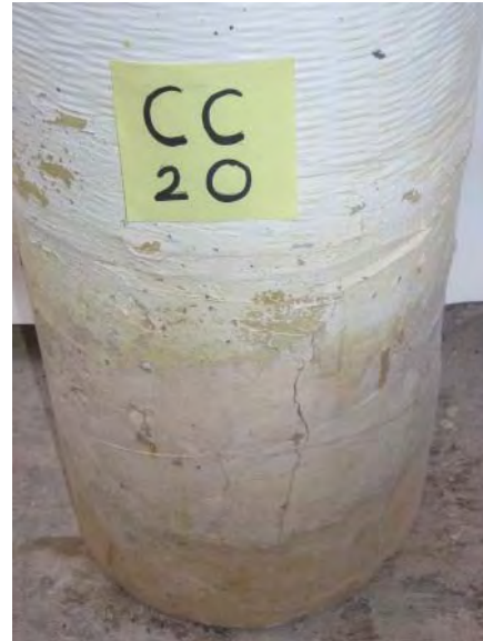
Crack over rebar A in unwrapped region.
