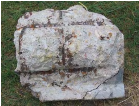
Lower areas of embedment of bars A and B. Note the repair material visible in lower right corner.
