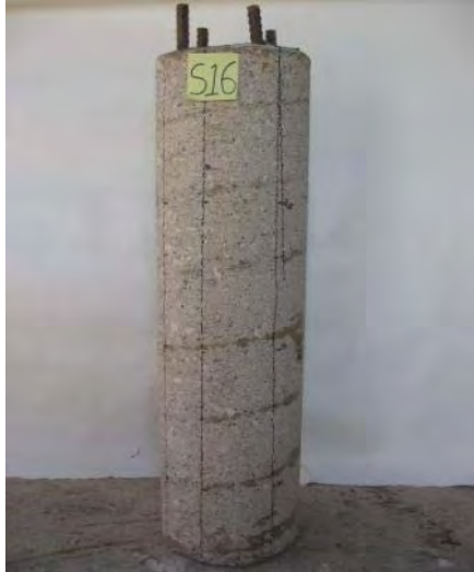
Cylinder S16 with wrap removed.
