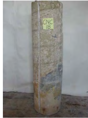
Repair patch and rust stains over rebar D.
