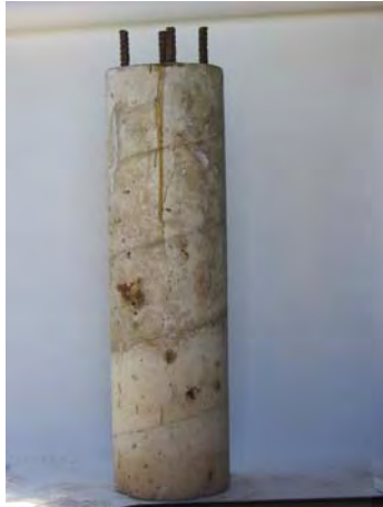
CNC15 full view with rebar A in front.
