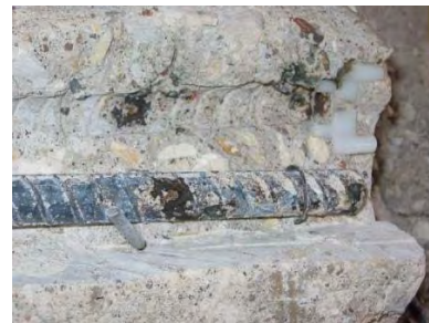
Heavy corrosion at 4 in. above bottom on rebar C
