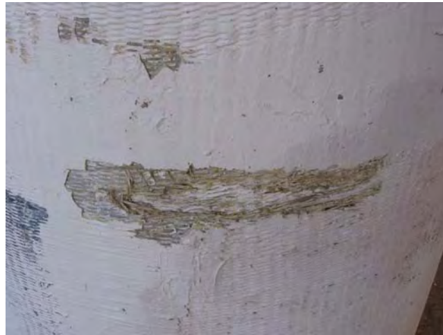
Figure 4.7 Damage on the upper layer of FRP wrap, Structure 7
