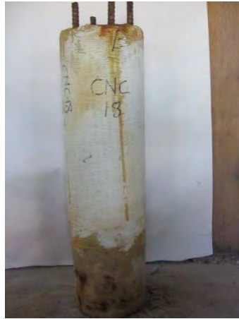
Cylinder CNC18 wrapped over top 24 in. Rust stains visible in unwrapped region.
