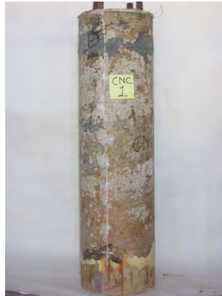
Cylinder CNC1 after removal of wrap.
