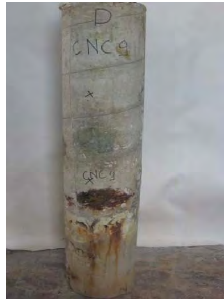
Rust stains and unconsolidated parts over rebar D.
