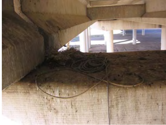
Figure 4.8 Location of embedded probe in Structure 8
