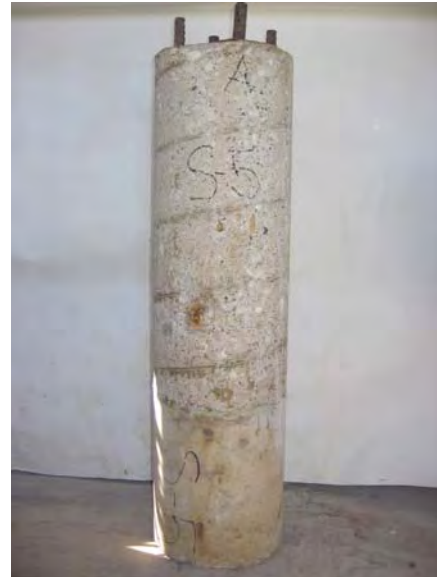
Cylinder S5 after removal of wrap.
