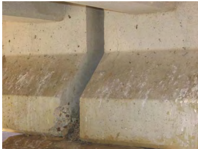
Figure 4.9 Cracking and Spalling of concrete at the end of girder, Structure 8
