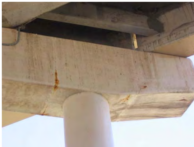
Figure 4.4 Rust staining on bent, Structure 1
