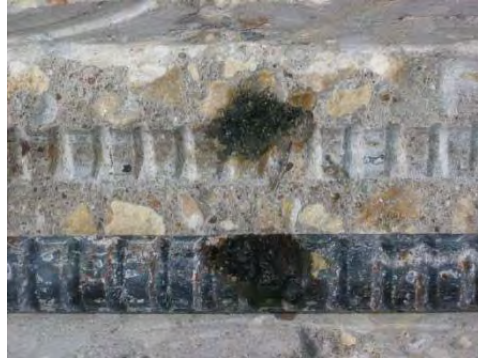
Heavy localized rusting on rebar A.
