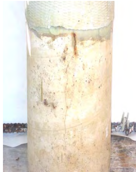
Crack over rebar C, starting where the wrap ends.
