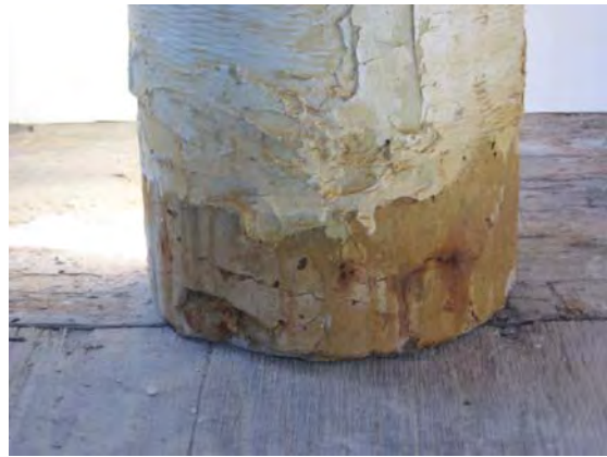
Detail of cracks and rust stains in unwrapped.
