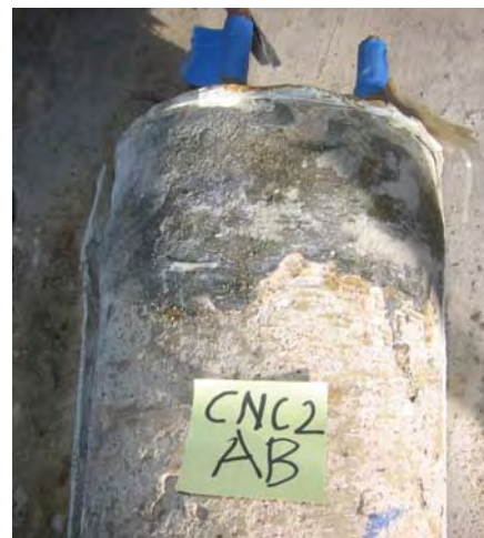
Trapped moisture under the wrap.
