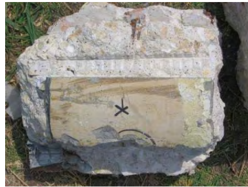
Areas of embedment of bars C and D. Corrosion did not take place due to presence of repair material.
