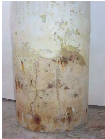
Crack and rust stains over rebar A.
