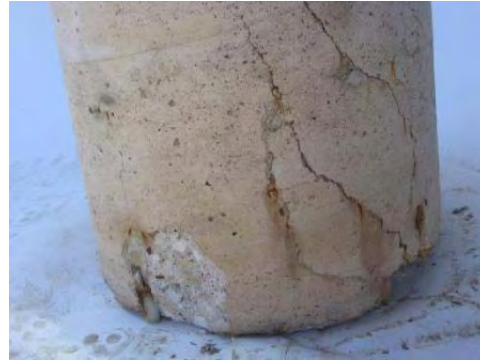
Spalling and cracking at bottom of Area AD.
