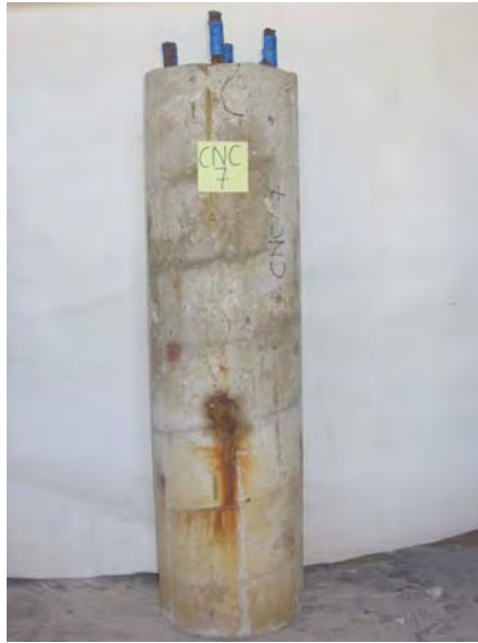
Cylinder CNC7 with large rust stain over rebar C.
