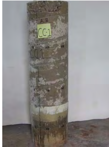
Cylinder CC1 after removal of wrap. Top 3 in. not consolidated properly.
