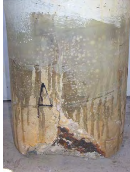
Detail of unwrapped region over rebar A.
