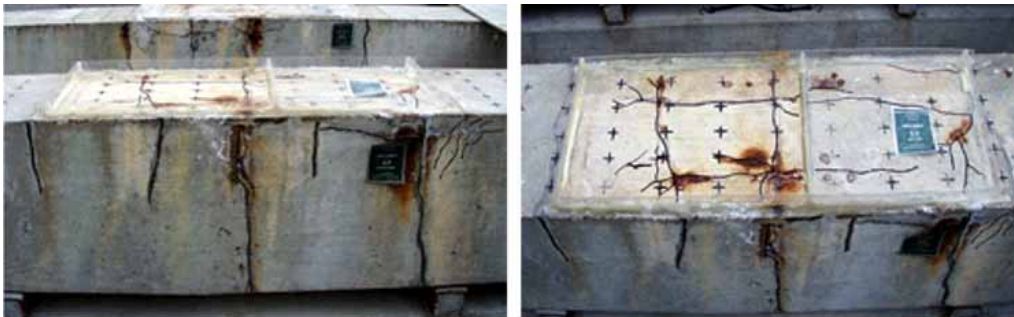
Lateral (South) View
