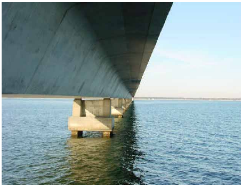
Figure 2.7 The Mid-Bay Bridge, Florida 16
