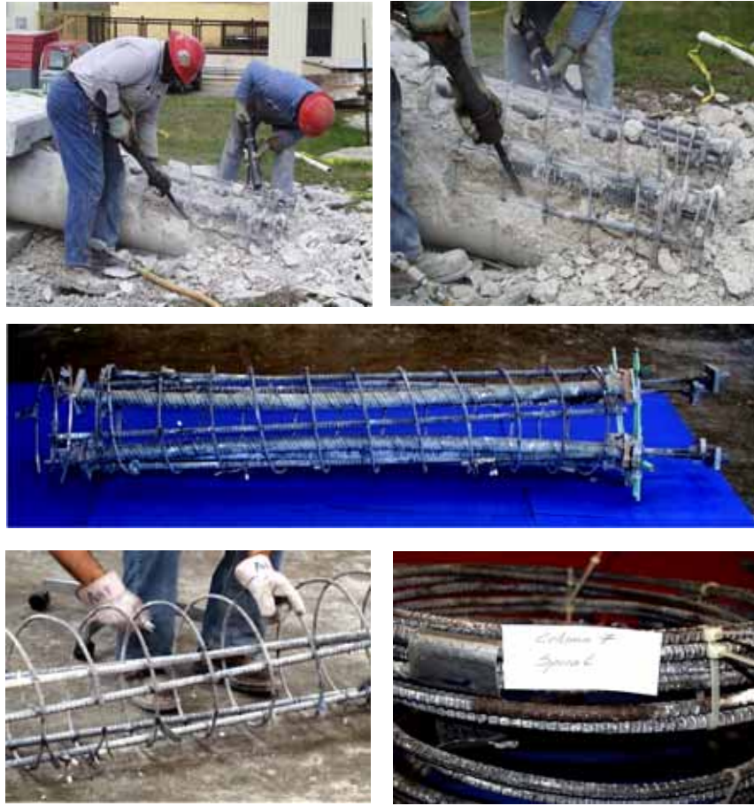
Figure 3.16 Column concrete Removal and Reinforcement Dismantling 37
