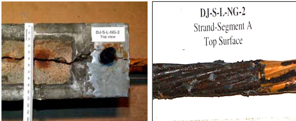
Figure 3.19 Example of Longitudinal (Splitting) Crack in Macrocell Specimen 83
