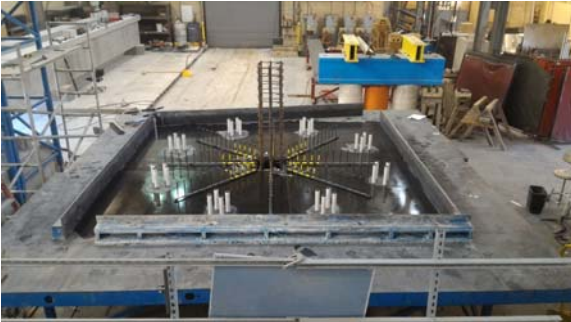
Fabrication of slab-column connection using circumferential stud rail configuration
