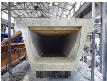
One hobo house available for rent. Minor cracking in the walls. Inquire in Office 202.
