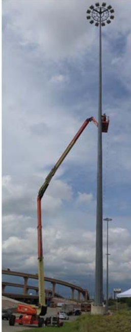
Researchers work to instrument a selected HMIP in Laredo.
