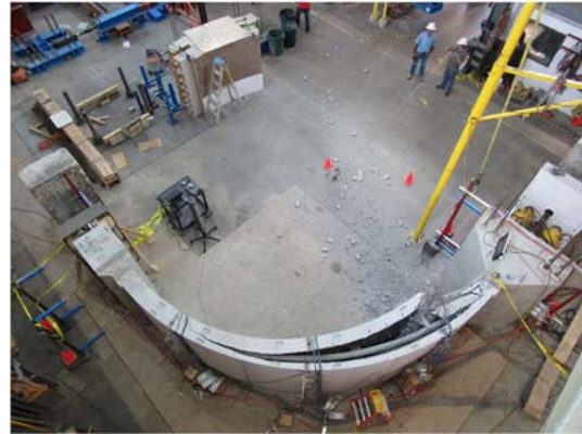
The third specimen after the failure
